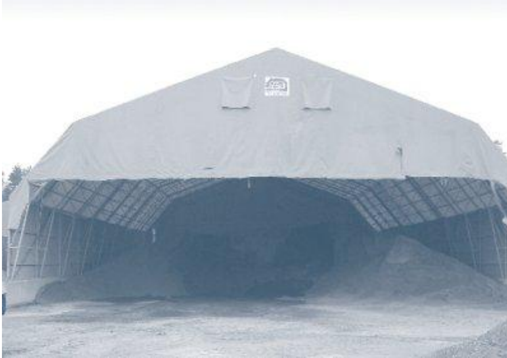
Figure 3 Kolo Veidekke Covered RAP Storage
