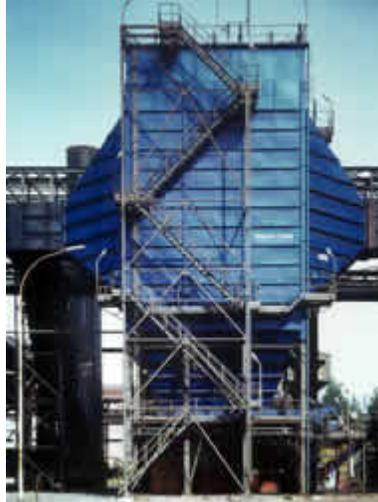
**Figure 2.1: Precipitator used to Control Emissions from a Wood Fired Boiler**
