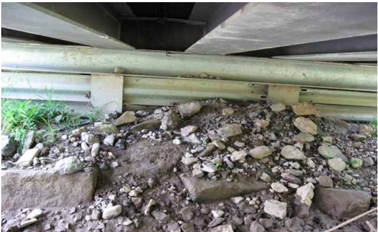
Figure 3.12: Conditions at the Bottom of Peel Tree Bridge
