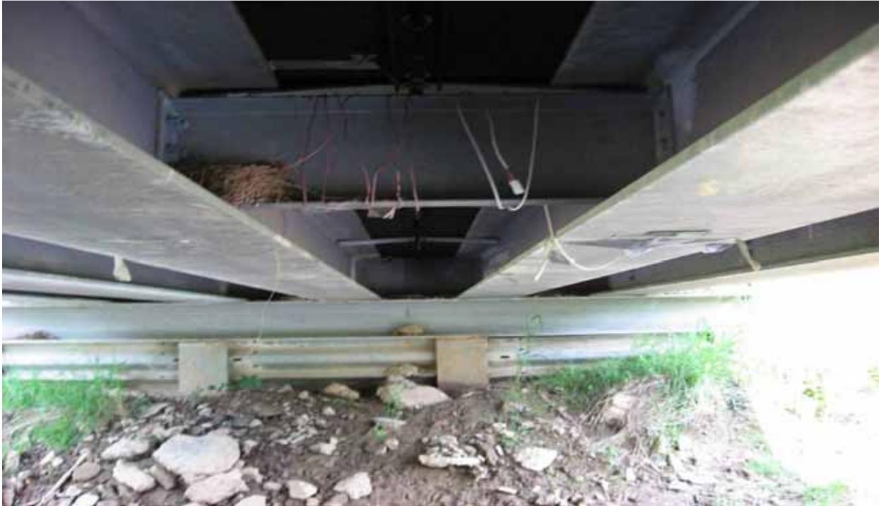
Figure 3.13: Bird Nest on the Diaphragm
