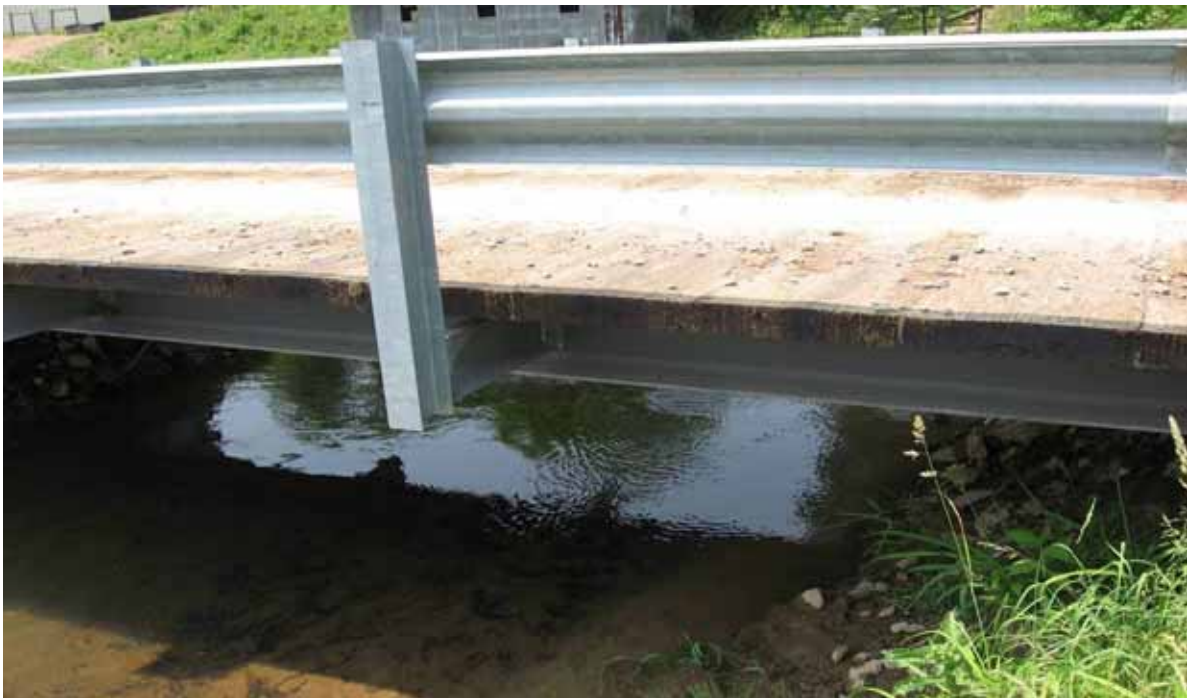
Figure 3.10: Guardrail Condition on Peel Tree Bridge
