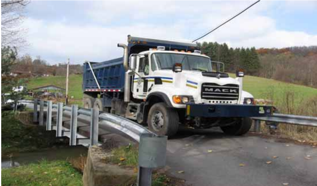
Figure 3.4: Static Live Load Test of Hackers Creek Bridge
