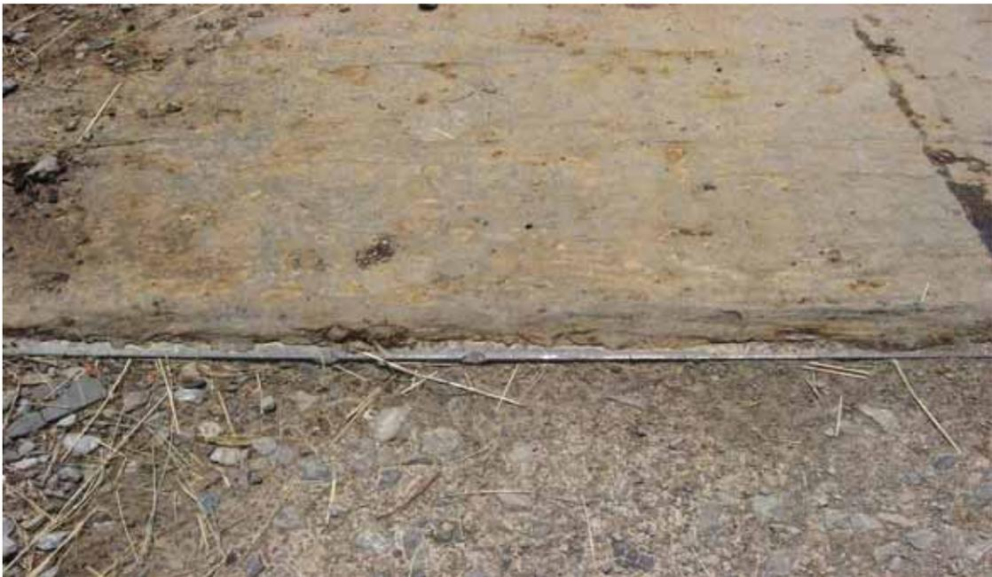
Figure 3.8: Parallam Deck Rolling on Peel Tree Bridge
