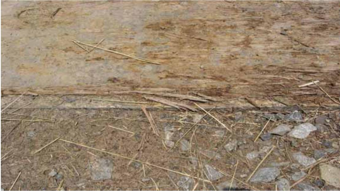
Figure 3.7: Parallam Deck Chipping on Peel Tree Bridge
