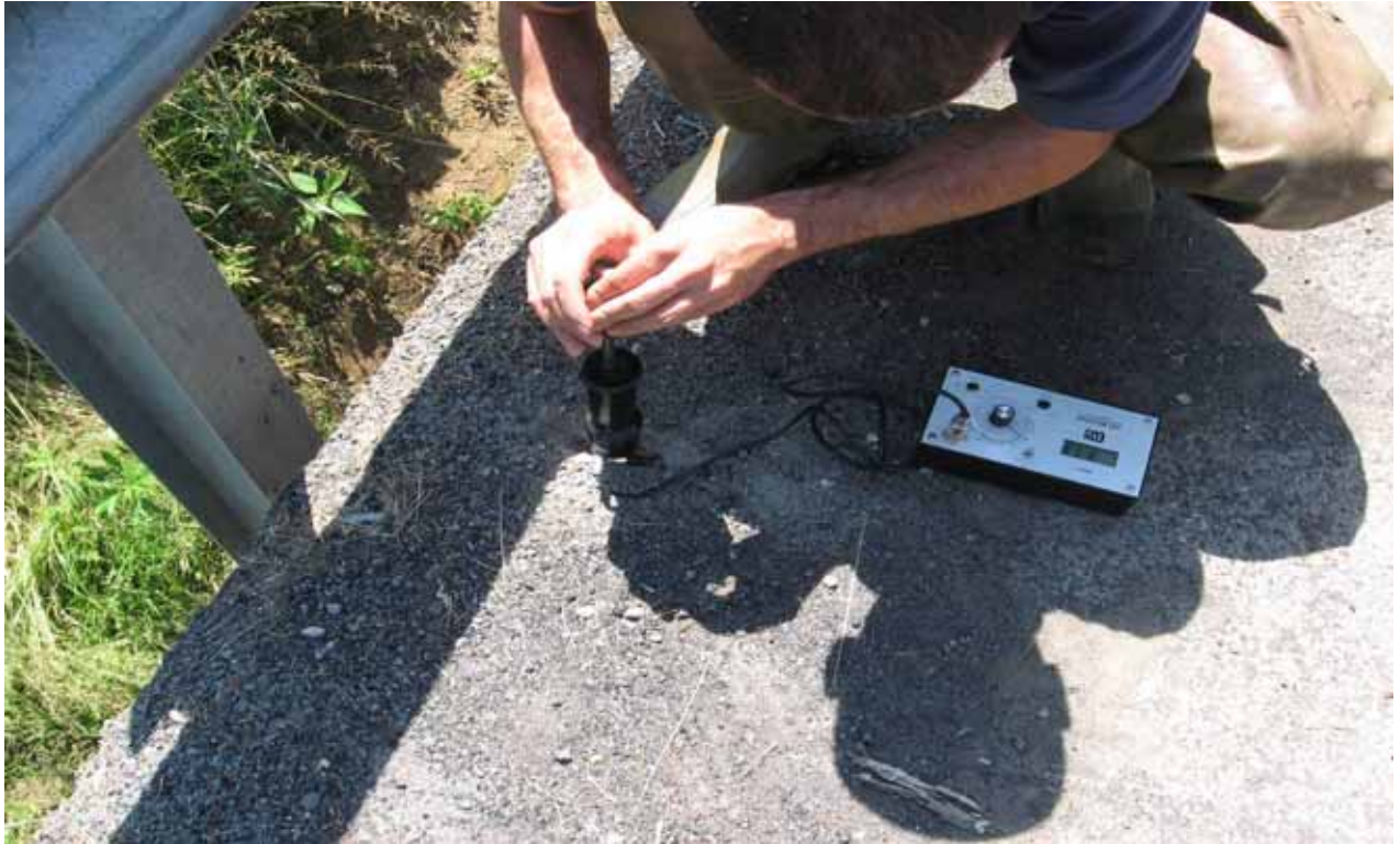
Figure 3.20: Taking Deck Moisture Content Readings on Hackers Creek Bridge
