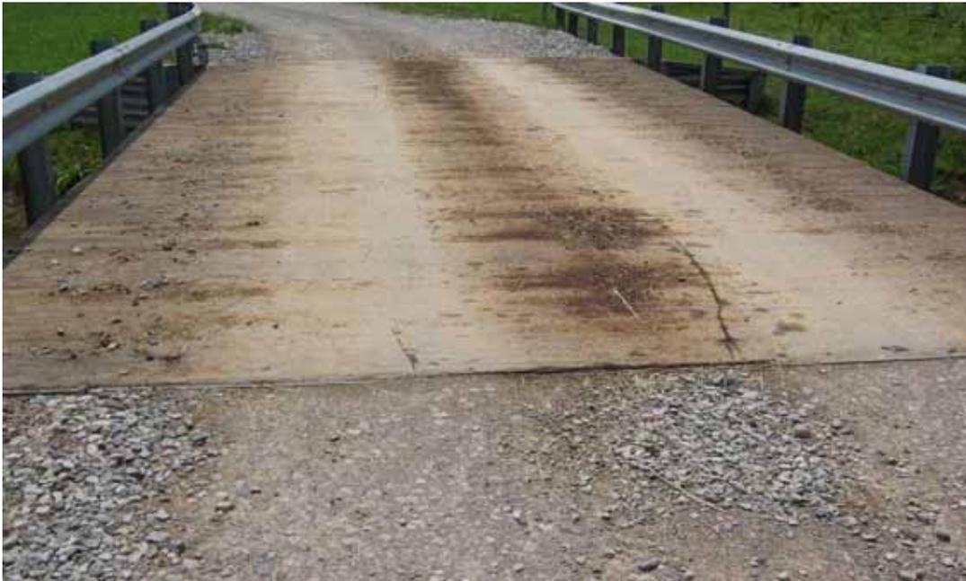
Figure 3.6: Wheel Path Rutting of the Deck on Peel Tree Bridge
