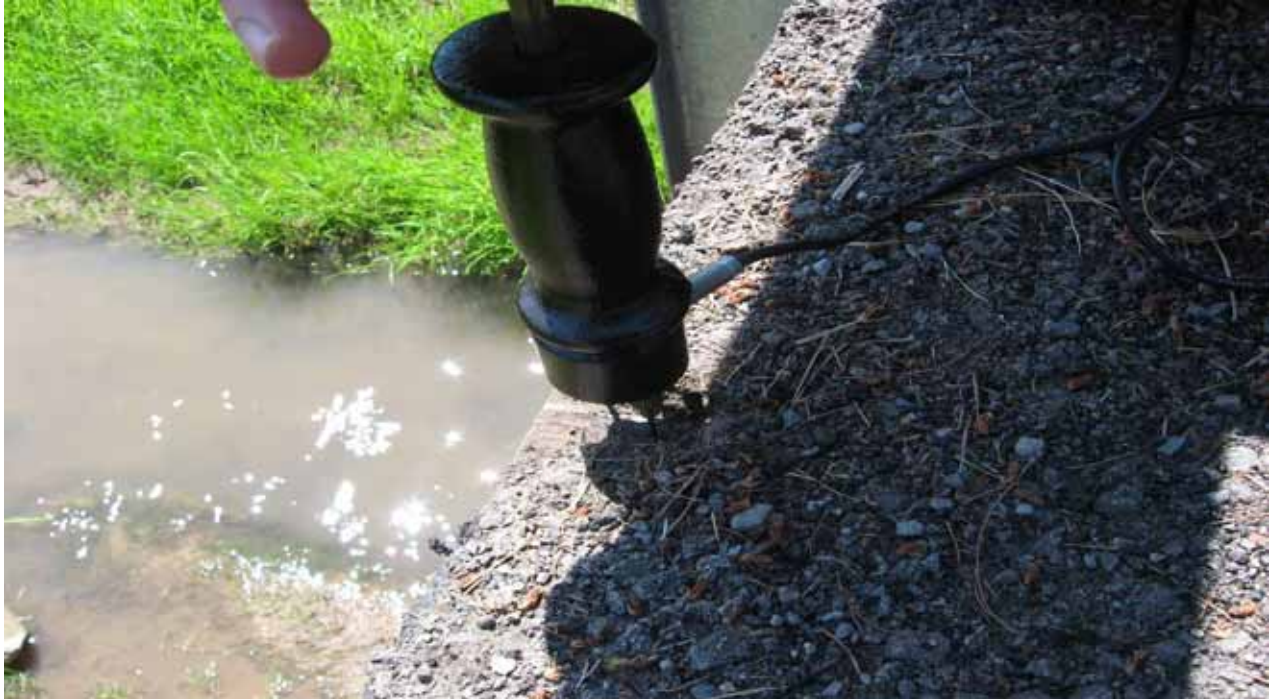
Figure 3.21: Taking Deck Moisture Content Readings on Hackers Creek Bridge
