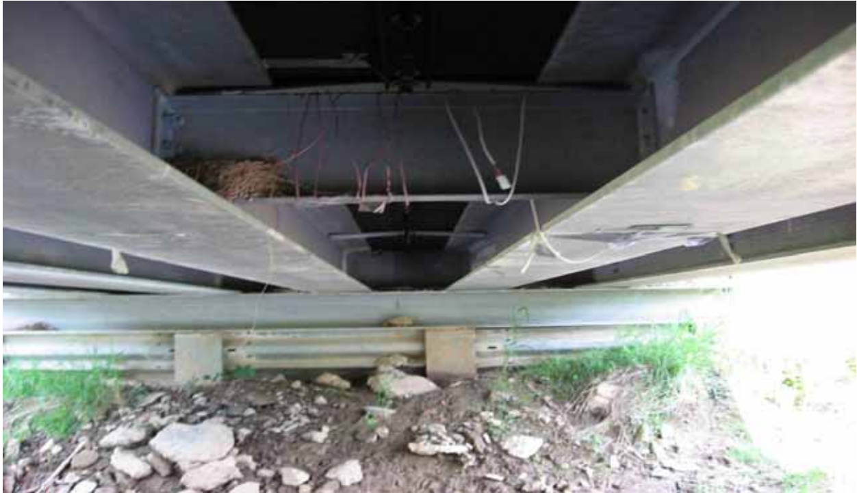
Figure 3.13: Bird Nest on the Diaphragm
