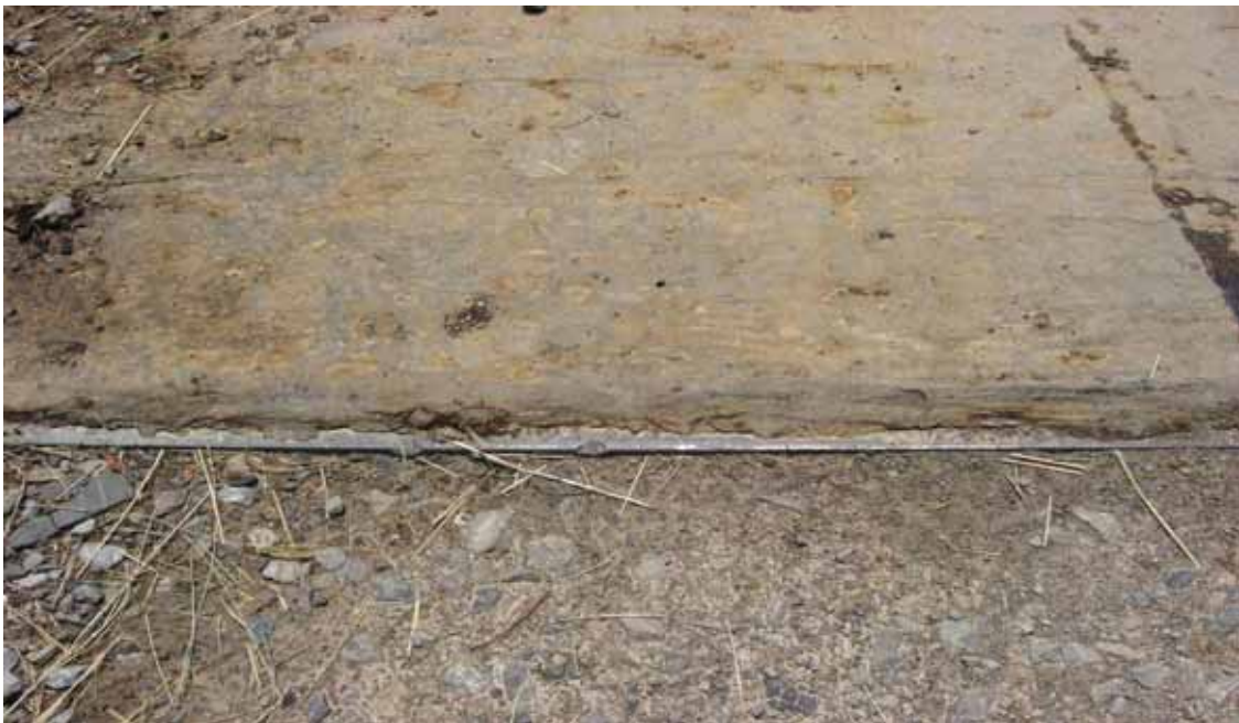
Figure 3.8: Parallam Deck Rolling on Peel Tree Bridge
