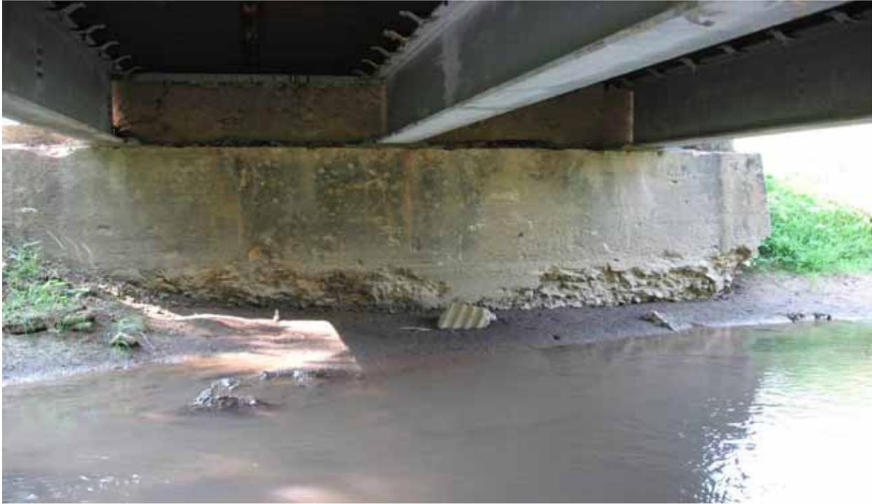
Figure 3.19: Disintegration of Concrete on the north abutment
