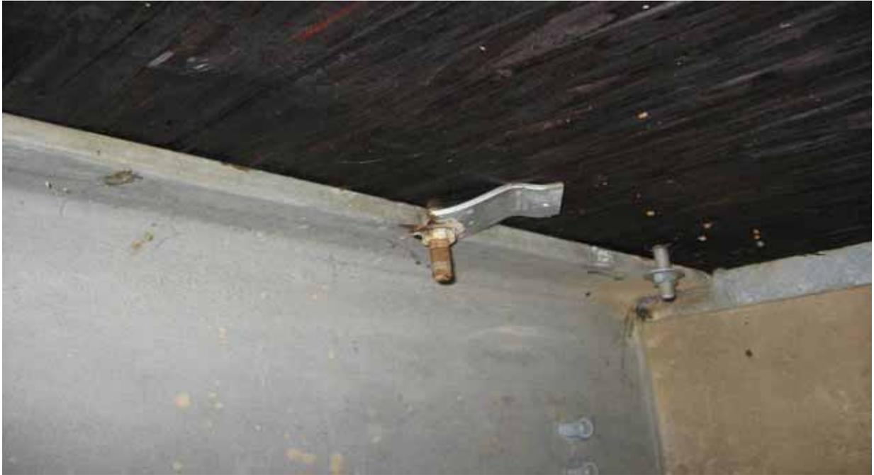
Figure 3.16: A Failed Stringer to Deck Connector on Hackers Creek Bridge
