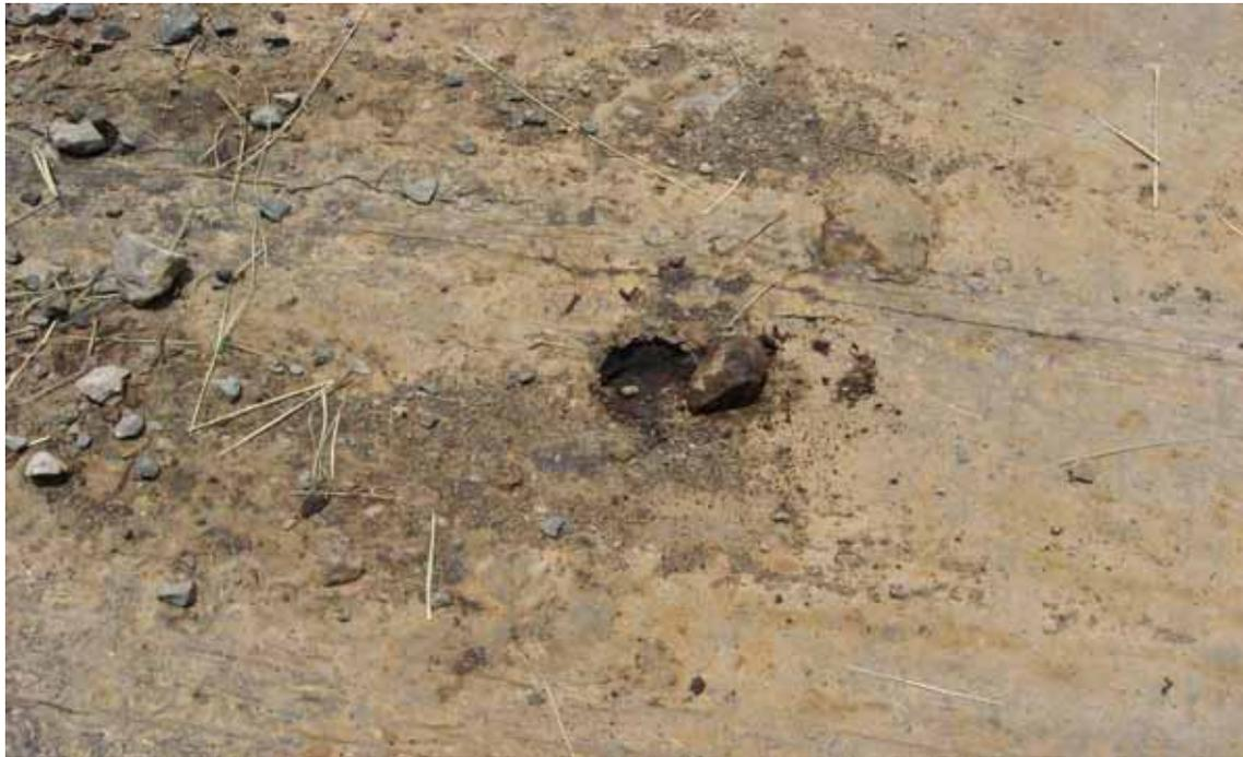
Figure 3.9: Indentation in the Deck Due to Gravel Driven in by the Traffic
